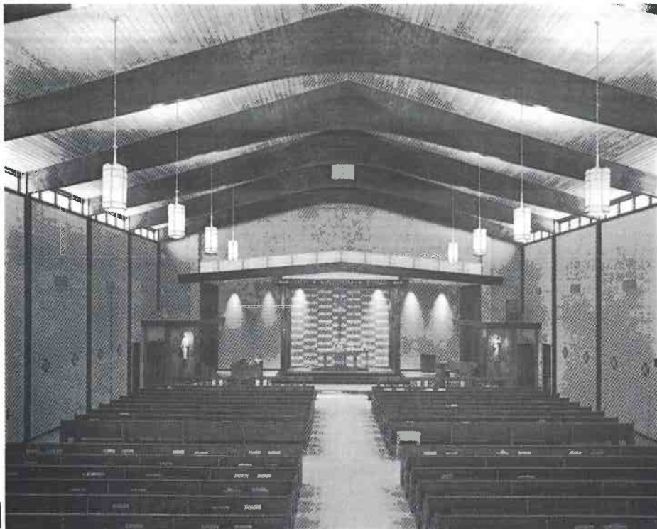
The original interior of St. Peter's Church, 1964.
