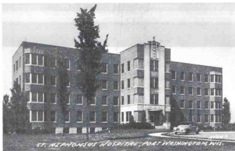
St. Alphonsus Hospital, 1941, before addition.
