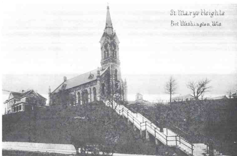
The newly completed cement stairway to St. Mary's - 1911
